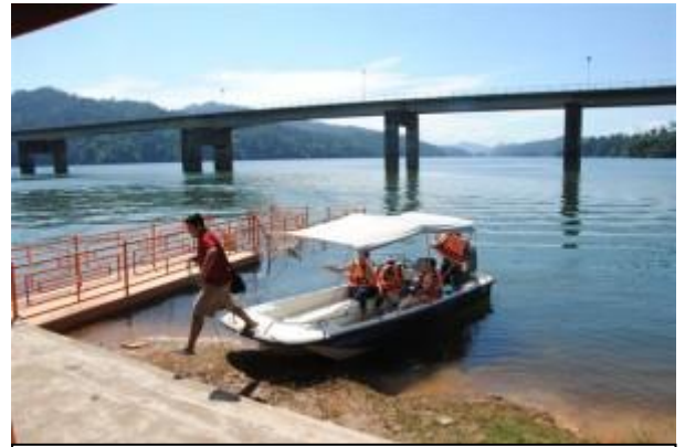
Banding Island's Useless Jetty
